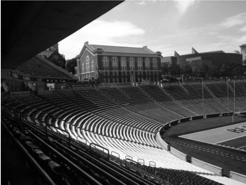
Figure 1: Stairway into Nippert Stadium
